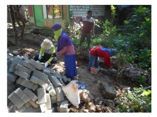
The third step is, applying cement and sand mixture on the bricks, to form the drainage wall.
