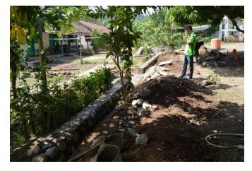
The embankment we built is 60 meters along the villagers' yard. It needs 2 trucks of sands, 2 trucks of stones, 18 sack of cements, 2 roll of building thread, and 2 buckets. It takes 6 days to do this project, with
