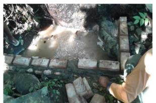
of sands, and tarpaulin to cover the water reservoir. First, campers with the help of villagers loaded all the materials into the water reservoir location. It takes 45 minutes – 1 hour to reach the location. Then we make the reservoir by arranging the bricks and cement to form wall, to hold the clean water.
