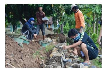
The water reservoir is needed so it will help the villagers in Liposos Paca to get more clean water. It takes 2 days to build the water reservoir, and we need materials such as 3 sacks of cements, 300 bricks, 1 truck
