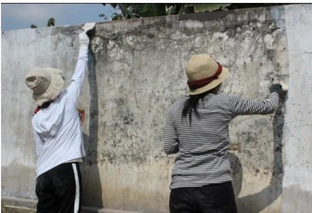
We removed cracked bricks on the wall and covered with cement as new wall surface.
