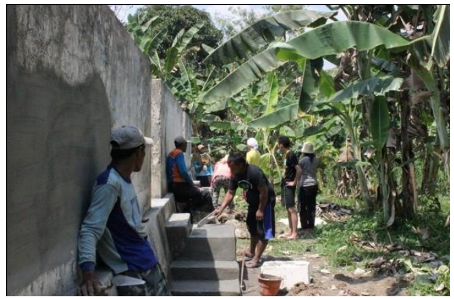
We removed cracked bricks on the wall and covered with cement as new wall surface.
