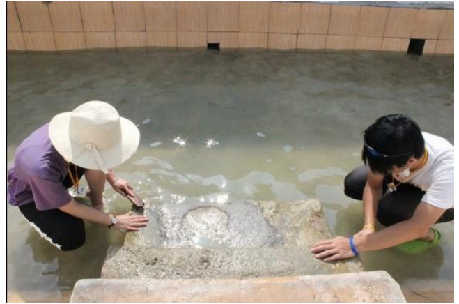
Cracked areas were patched by cement and steps into the bath also repaired.
