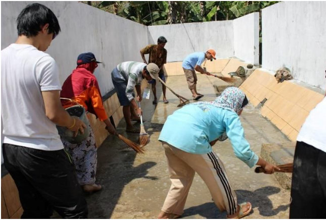
Cracked areas were patched by cement and steps into the bath also repaired.
